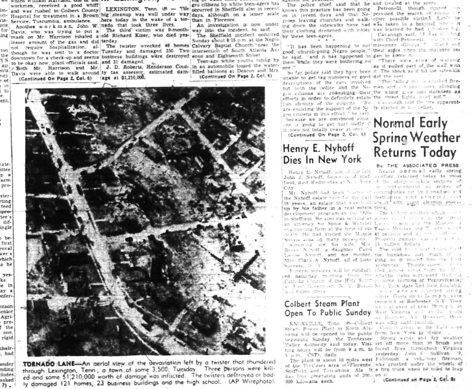
TORNADO LANE —An aerial view of the devastation left by a twister that thundered through Lexington, Tenn., a town of some 3,500. Tuesday. Three persons were killed and some 51,210,000 worth of property was inflicted. The twister destroyed or badly damaged 121 homes, 23 business buildings and the high school. (AP Wirephoto).
