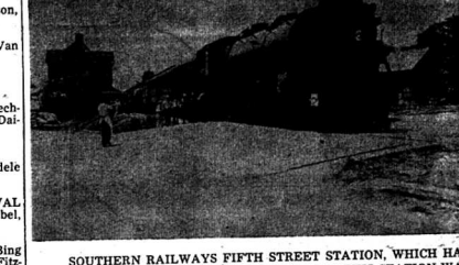
SOUTHERN RAILWAYS FIFTH STREET STATION, WHICH HAS BEEN ABANDONED AND TRACKS REMOVED, AND IT IS A SAD SIGHT TO OLD TIMERS TO SEE IT GO.
